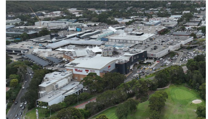
Aerial view of Westfield, Warringah Mall. Largest retail floor plate of 3-4 storeys with large parking areas.
