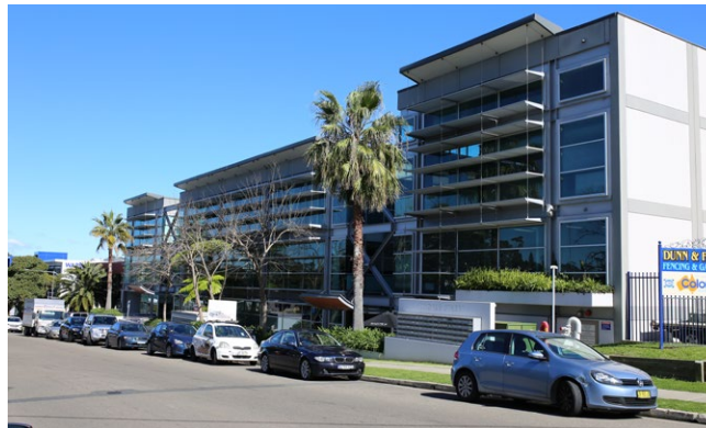
View of 20 Dale Street, existing 3 storey office building within General Industrial zone providing a range of services.
